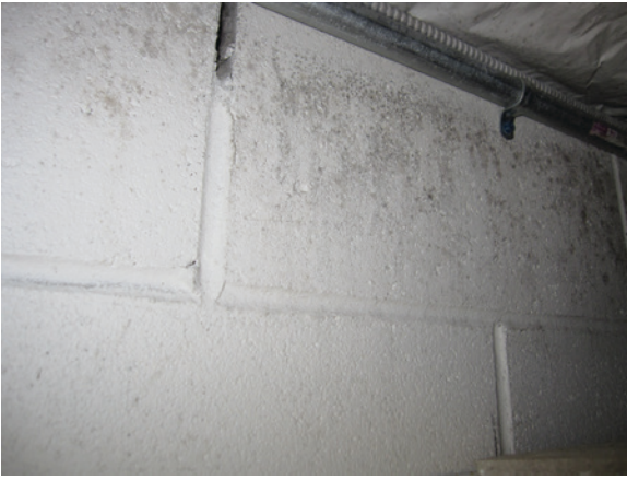
Figure 1-2 Mold growth on painted concrete masonry. The cool masonry wall separates a classroom from an ice rink. Humid air in the classroom provides moisture that condenses on the painted surface of the masonry. That moisture allows mold to grow on the paint film.
